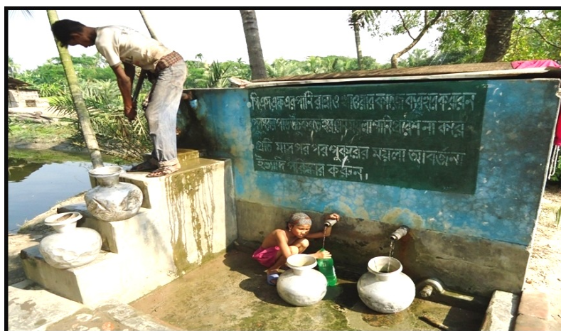
Figure 2: Existing water supply facilities in Shamnagar Upazila
